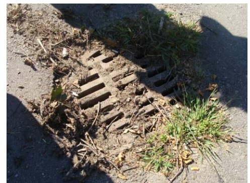
Stormwater catch basins require regular maintenance in order to remain clean and clear of debris, trash, and sediment.
