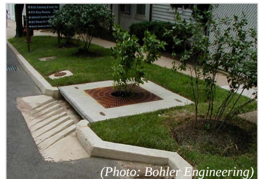
(Photo: Bohler Engineering) Tree box filters are recommended to reduce pollutants draining to all storm drains along Madison Avenue.
